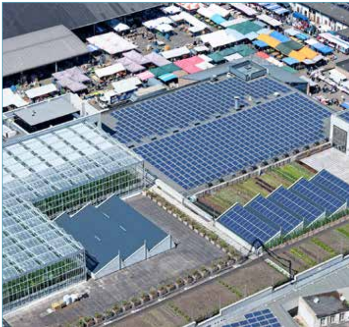
figure 7: PV panels and urban agriculture on the Foodmet building, 2017 (Abattoir nv)
