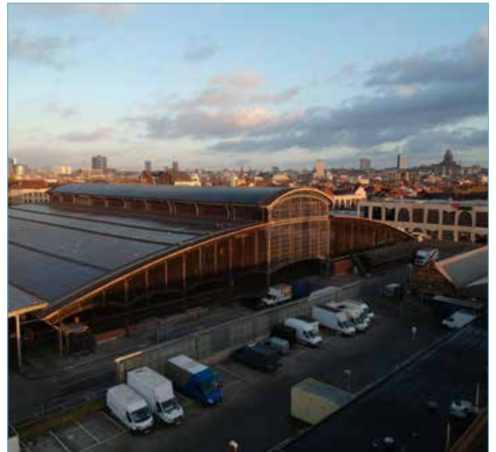
figure 8: PV panels on the covered market, 2021 (Abattoir nv)
