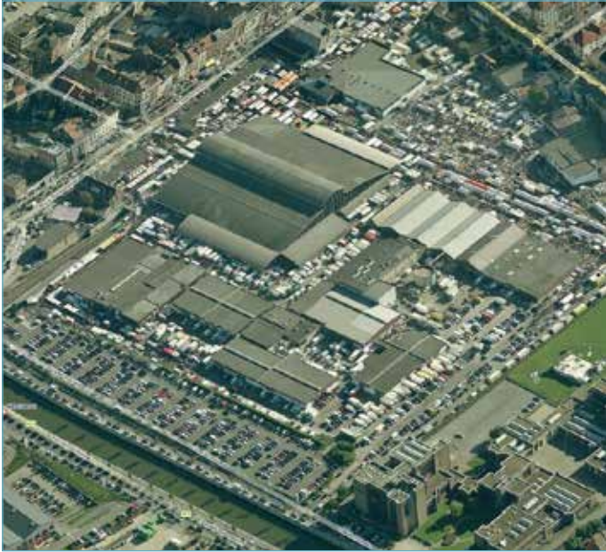
figure 3: aerial picture of the Abattoir site before the start of the redevelopment (Abattoir nv)
