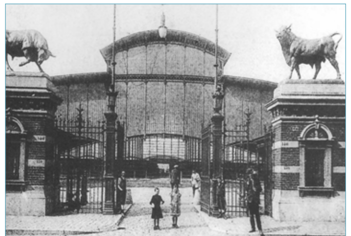
figure 2: picture of the Abattoir market hall in the 19 th century (Abattoir nv)
