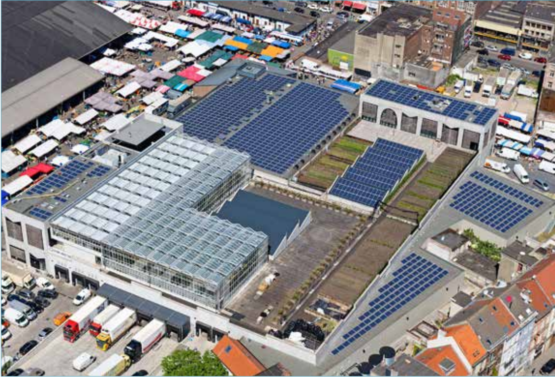
figure 21: aerial view of the Foodmet project, with the photovoltaic installations (and the aquaponic and other urban agricultural activities) clearly visible. (Abattoir nv)
