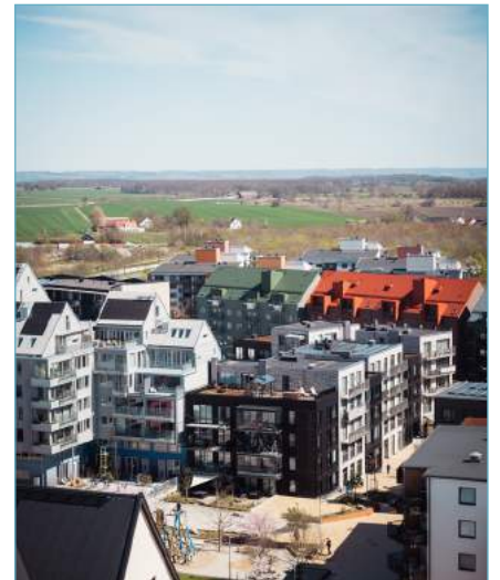
figure 6: a completed part of the Brunnsög project (City of Lund)
