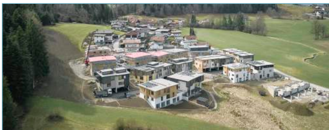
figure 11: The Sonnendorf construction site in April 2022 (David Schreyer)
