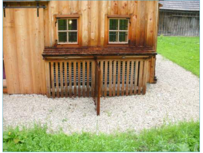
figure 15: an installed heat pump at one of the houses (Kleboth & Dollnig)
