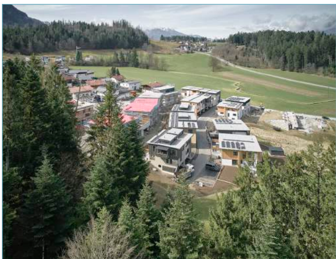
figure 12: PV panels on the roofs of the completed houses, April 2022 (David Schreyer)
