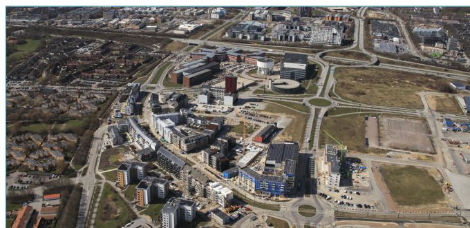
figure 3: the Brunnskög PED under construction (City of Lund)
